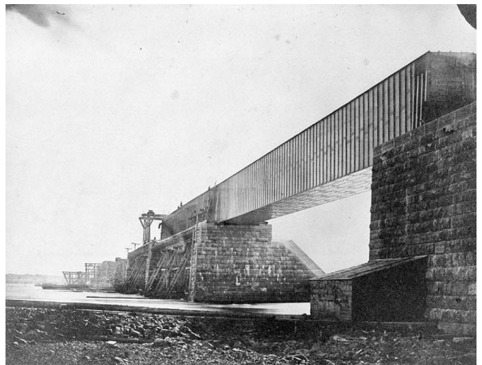
The Victoria Bridge under construction, c. 1858-1860
